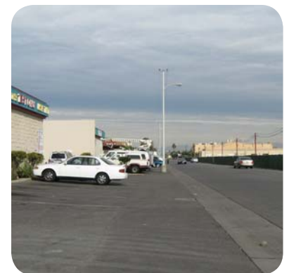
Portions of Moran Street lack curb, gutters, and sidewalks.
