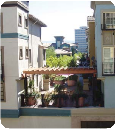
Common outdoor space may include courtyards, plazas, or similar spaces open to the sky.
