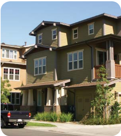
Windows, overhangs, fixtures and other details reduce a building's scale.
