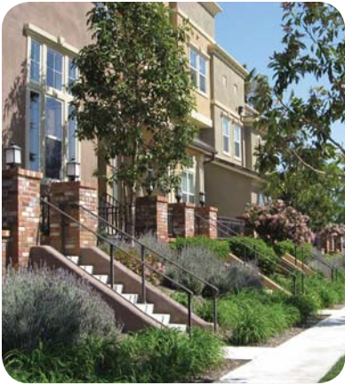
Direct access to individual residential units should be elevated from the street.
