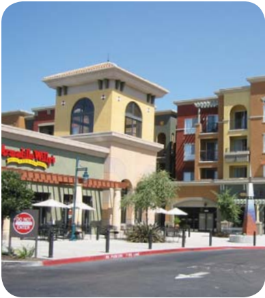
Multiple buildings in a mixed-use development should vary in height.
