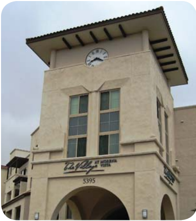
A taller, prominent rooftop element conveys the feeling of importance.
