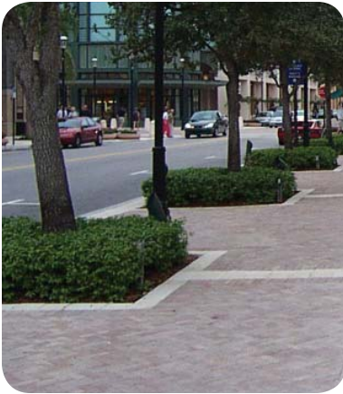
Paving treatments provide clear identification of pedestrian walkways.
