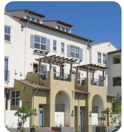
The top floors of multi-family buildings should be set back to make them appear more human in scale.
