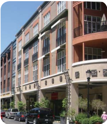
Neutral earth tones should be used as the predominant color for exterior walls.
