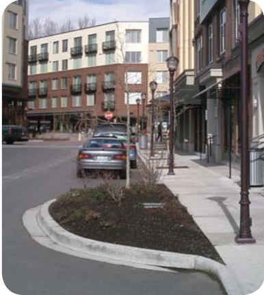
Bulb-outs are a traffic calming technique used to improve the pedestrian experience.
