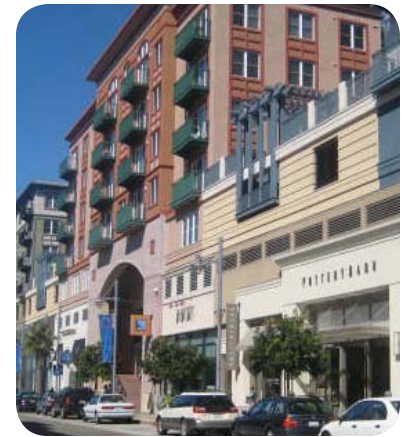
Major utilities and pull-boxes should be out of the line of sight.
