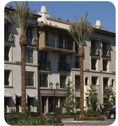
Recessed windows provide depth to a building's exterior.
