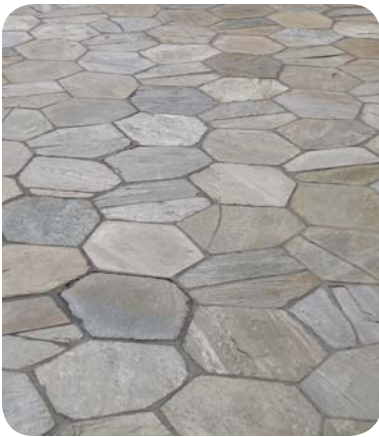
Natural stone pavers should be used to provide clear identification of pedestrian walkways.
