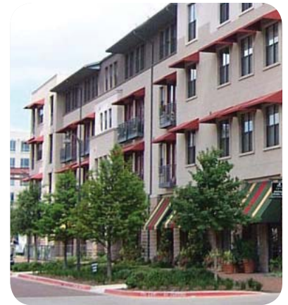
Deciduous trees help with solar control during summer and winter on southern and western facades.
