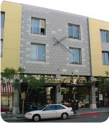
Creative use of materials can enhance the appearance of a building.
