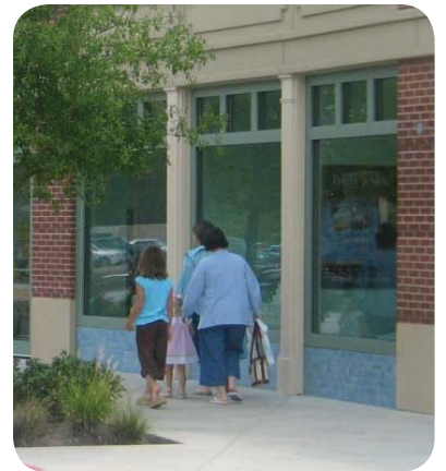
A bulkhead of approximately 24 inches in height should be used below store windows.
