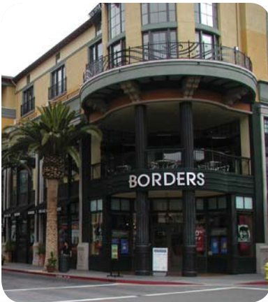
The use of prominent corner entries should be used at significant intersections.
