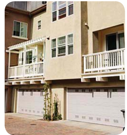
Garage doors should be recessed into, rather than flush with, the exterior wall.
