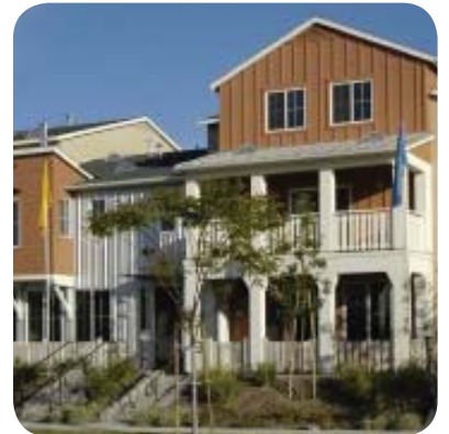
Long, unbroken facades can be avoided by using balconies, porches or other elements.
