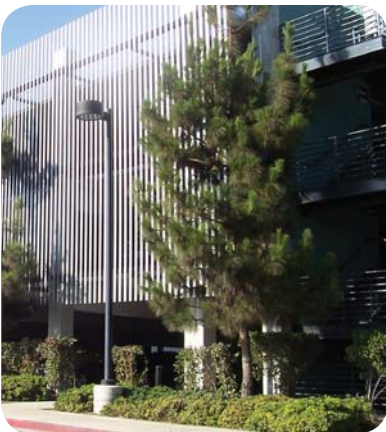
Parking structures shall be screened with vertical landscaping to soften their appearance.
