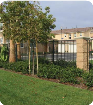
A design feature shall be provided along a wall or fence every 12 feet to add interest.
