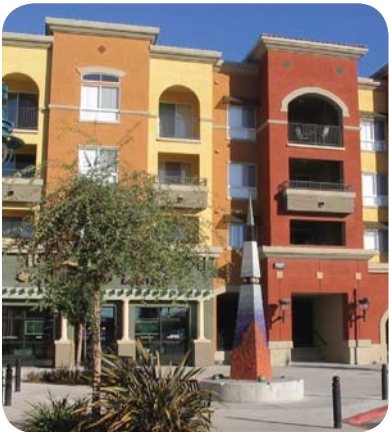
Variation in the wall plane helps to make the building appear smaller in scale.
