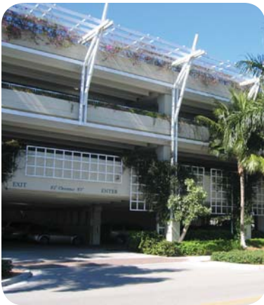
Parking structure exposed on all levels with landscape screening at the ground floor.
