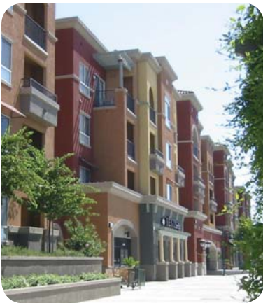
Smooth stucco and painted concrete and wood should be the primary exterior materials.
