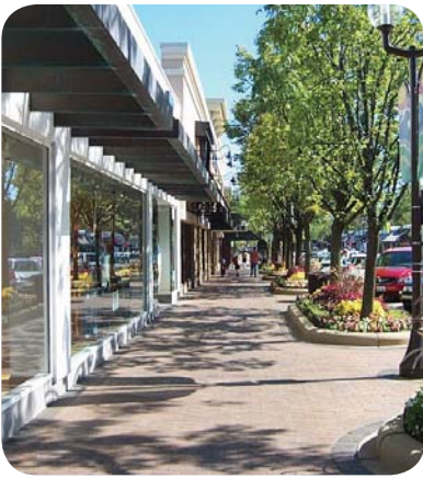
Appropriately scaled buildings, attractive storefronts, and wide walkways improve the pedestrian environment.
