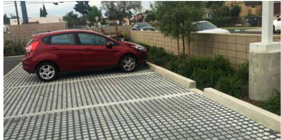
Permeable paving breaks up asphalt and can reduce the heat island effect.
