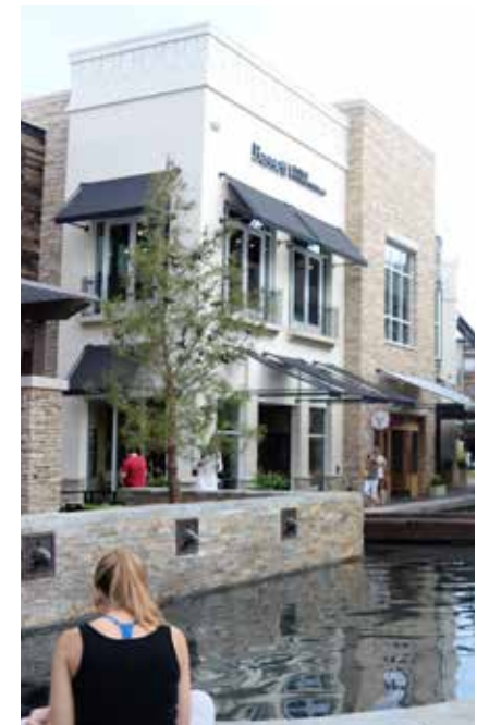
Careful building placement and thoughtful architectural design will create a sense of place at the Mall.
