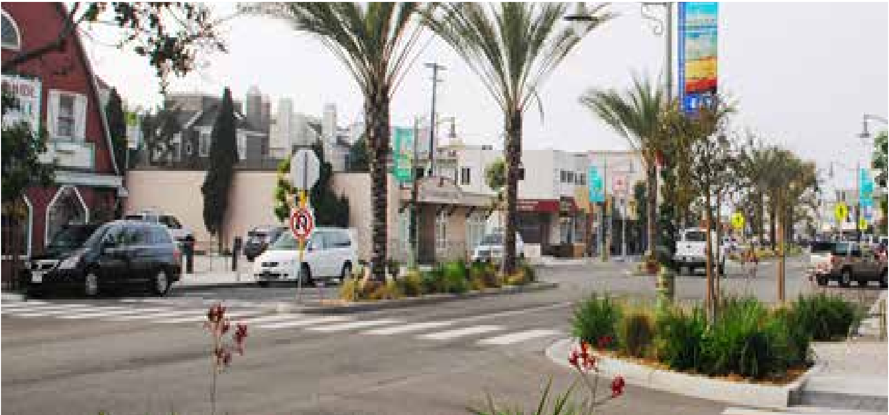
Bulb-out at crosswalks with high-visibility continental striping improves pedestrian safety by limiting exposure to vehicles.
