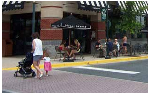
Paving treatments improve visibility of pedestrian crossing areas.
