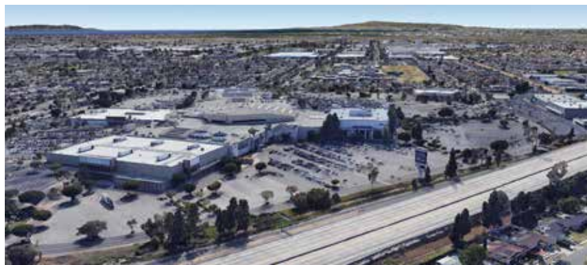
Existing view into the WMSP looking west from the I-405 Freeway.
