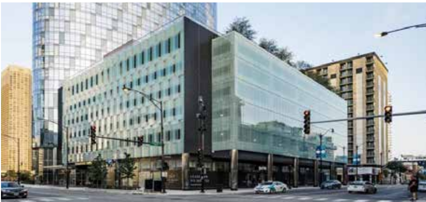
Parking structure with an integrated building facade and formal entry creates interest and uniformity with surrounding buildings.
