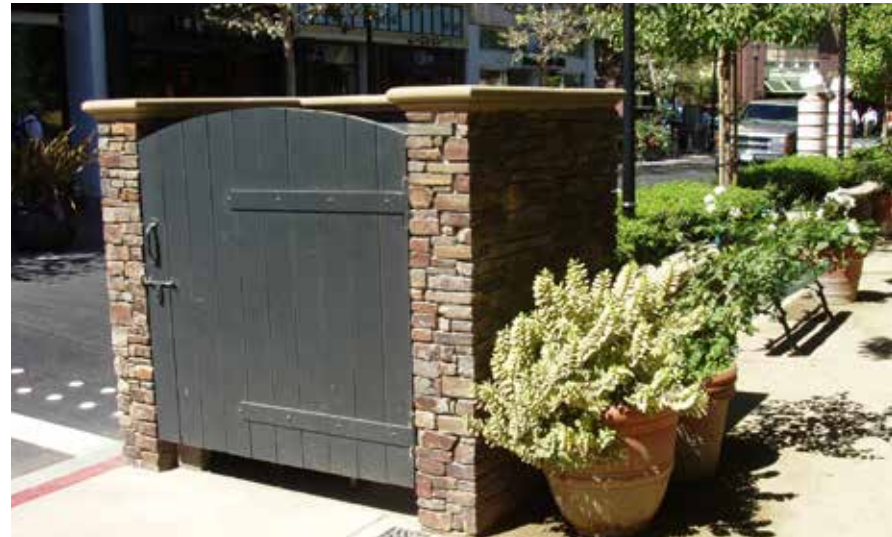
Using materials and design complementary of site disguises utilities.
