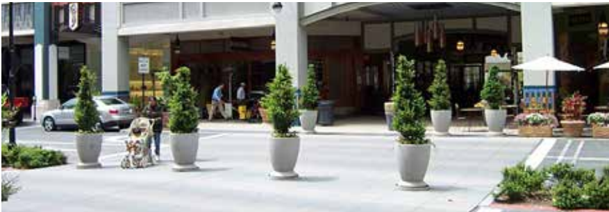
Raised planters in crosswalk for pedestrian safety and directing traffic flow
