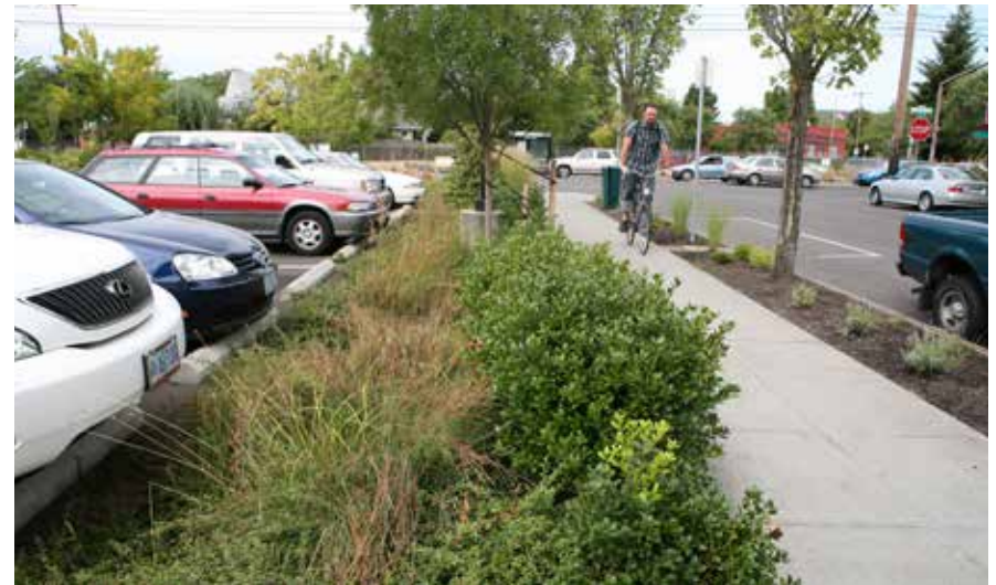
Biofiltration adds another benefit to medians by collecting and filtering water runoff from parking lots, helping to lower pollution and storm water.
