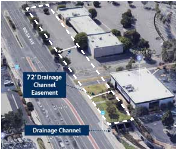
The drainage channel easement will be an opportunity to provide a unique frontage edge along Bolsa which may include open space and /or a frontage road
