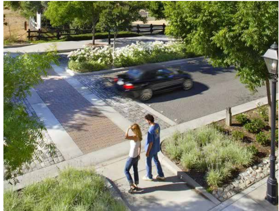
Permeable paving and landscaped bulb-outs help control water drainage around the site.
