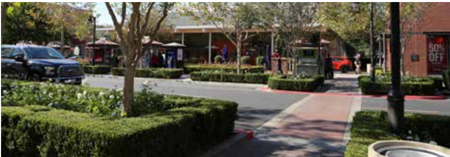
Change in paving and bulb-out bring driver awareness to crosswalk.
