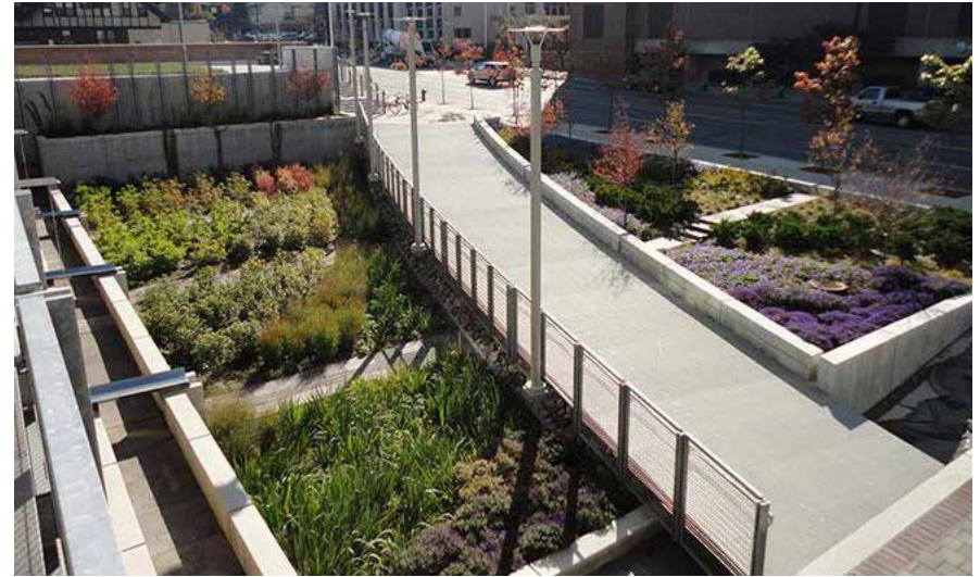
Rain gardens are an attractive use for collecting and mitigating water runoff around the site.
